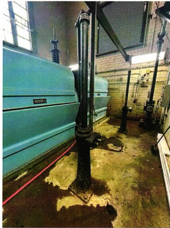
Figure 13 (Left): Sluice Gate #1 on Pump Side for Screen Channel #1 Figure 14 (Right): Sluice Gate #2 on Pump Side for Screen Channel #2
