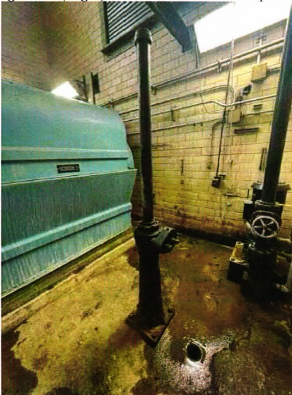
Figure 15 (Left): Sluice Gate #3 on Pump Side for Screen Channel #3 Figure 16 (Right): Sluice Gate #1 on River Side for Screen Channel #1
