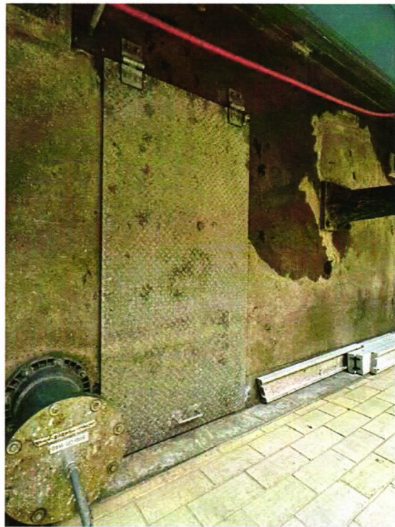
Figure 10 (Right):: Access Hatch that houses the interior stop log guide slot
