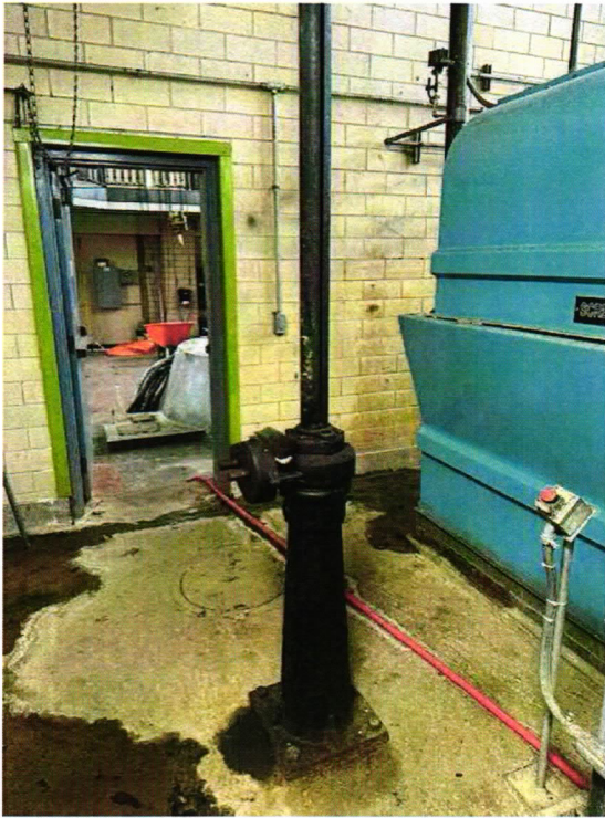
Figure 13 (Left): Sluice Gate #1 on Pump Side for Screen Channel #1 Figure 14 (Right): Sluice Gate #2 on Pump Side for Screen Channel #2
