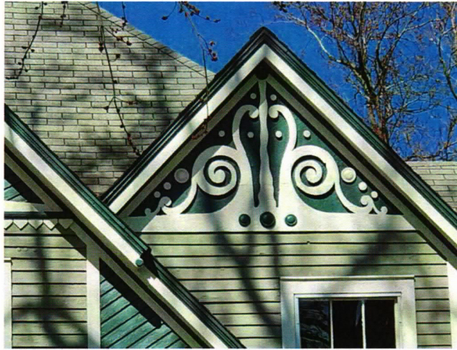
Brentwood S. Tolan House- detail of secondary gable of the façade (2022)
