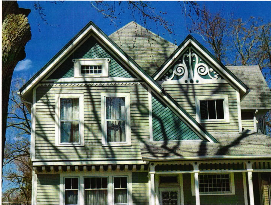
Tolan House, 316 W. DeWald Street; façade detail
