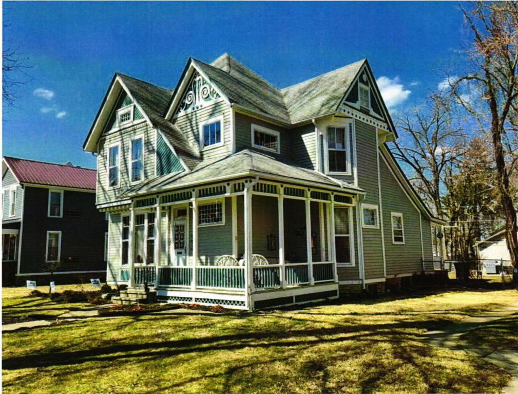
Tolan House, 316 W. DeWald Street; façade and east elevation
