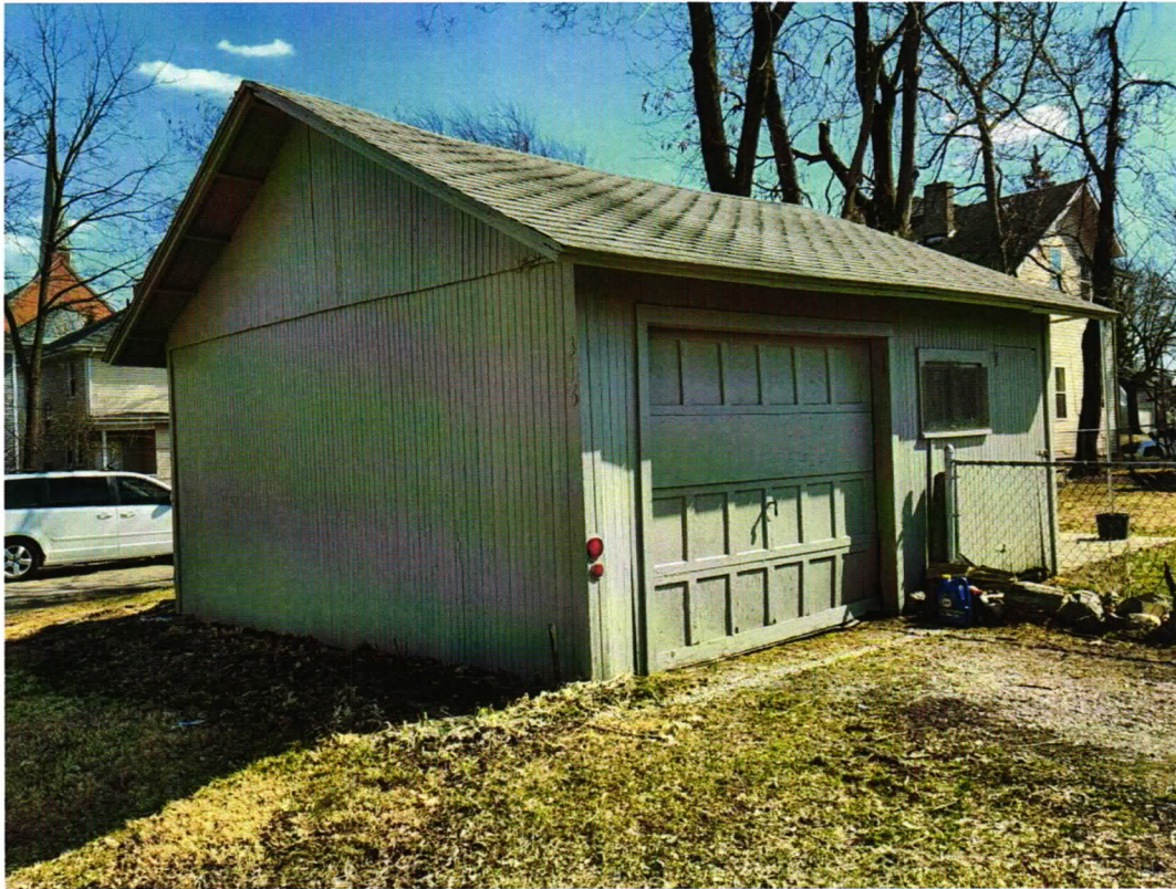
Tolan House, 316 W. DeWald Street (garage) All photos were taken in 2022
