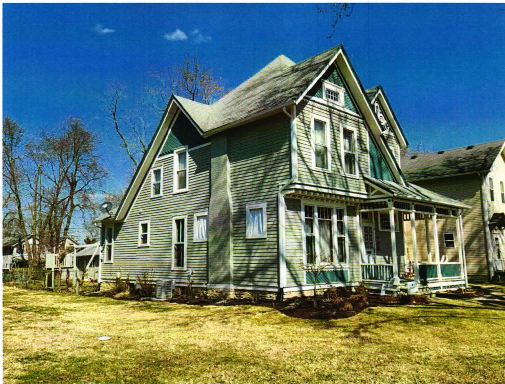
Tolan House, 316 W. DeWald Street; façade and west elevation
