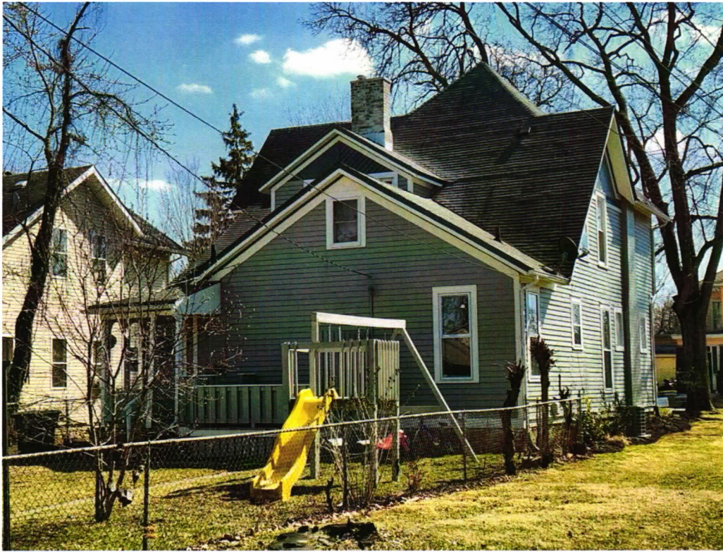
Tolan House, 316 W. DeWald Street; rear and west elevation
