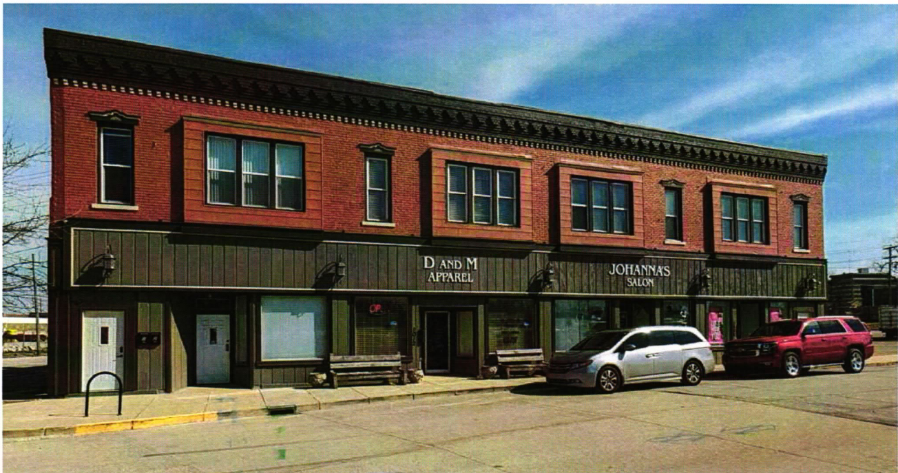
Hake Block Façade – Photo Taken 2/21/2024
