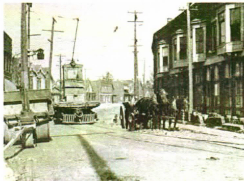
Above: Work motor 22, as it appeared in 1921, already had been reconstructed more than once; it would change again in 1929. Here it works on Wells Street in 1921. Bradley-Hansch Collection. Below: J.C. freight motor 841 was a reconstruction of FW-L 45. It later became IRR 726. Russ Powell is the motorman in this 1935 scene in Indianapolis. George Krumler Collection.
