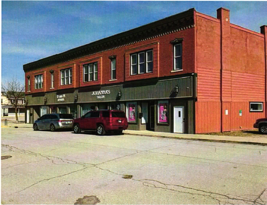
Façade and South Elevation
