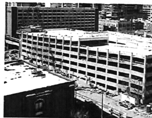
CIVIC CENTER PARKING GARAGE FORT WAYNE, IN OVER 200+ NEW PARKING SPACES
