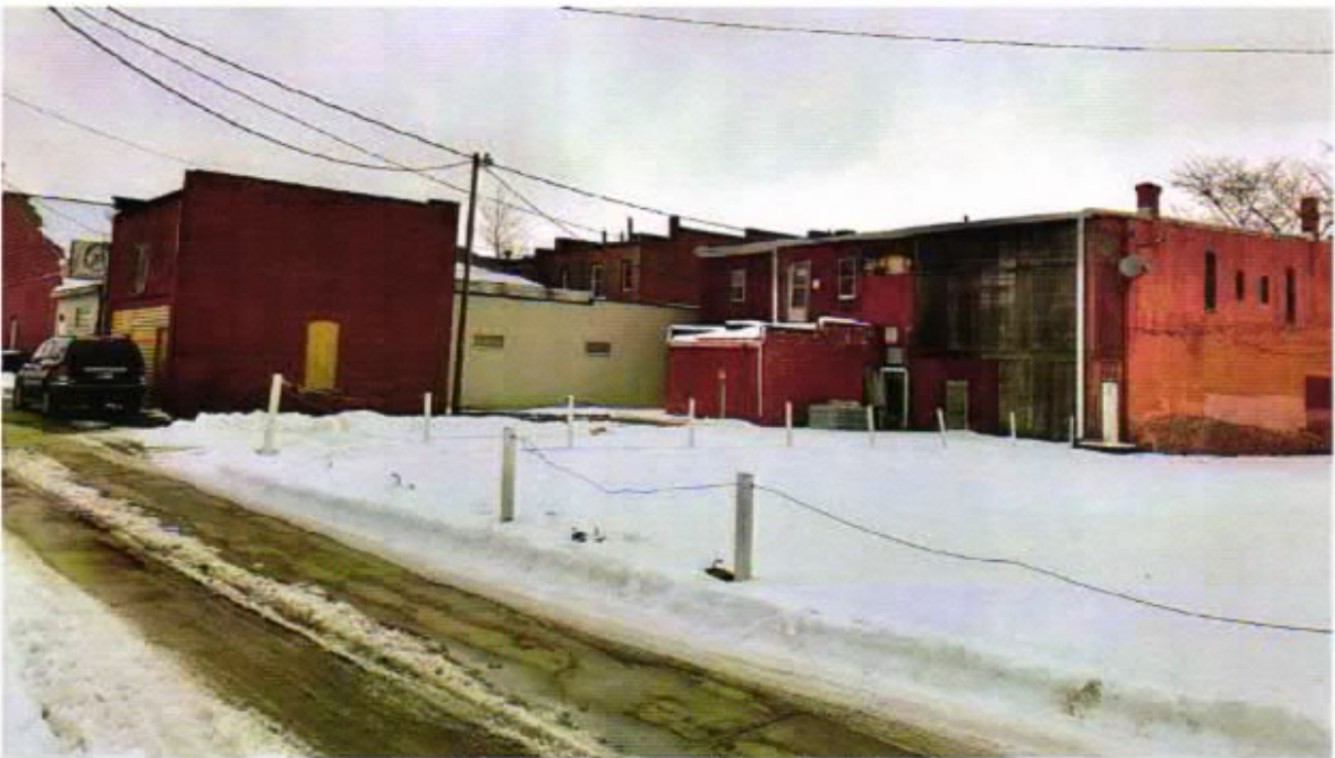
View from SW corner of district looking NE
