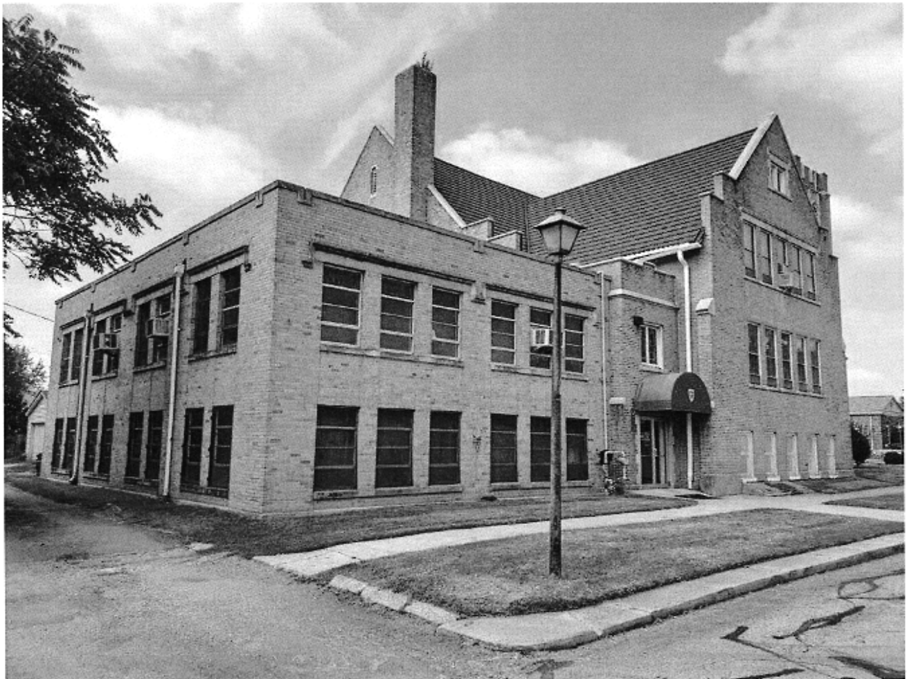
Calvary United Brethren—Turner Chapel AME Church, looking Northwest at the south and east elevations of the 1954 addition.
