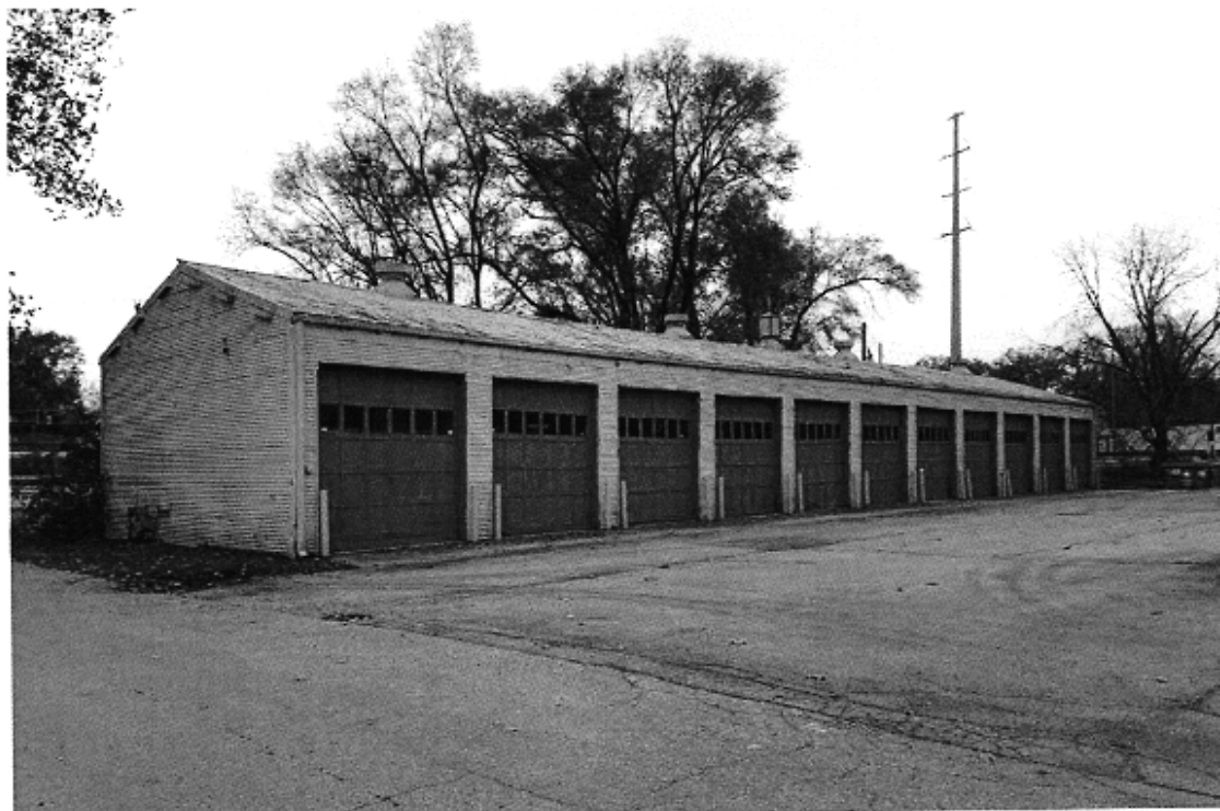
Charles F. & Mollie Centlivre House; Centlivre/Old Crown Brewery delivery truck garage, east and south elevations. Photo looking northwest.
