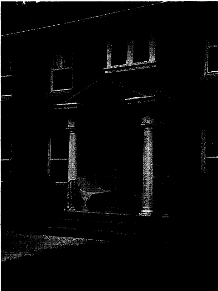
Dr. Robert and Susie McKeeman House, front porch, looking northwest; July 11, 2017.
