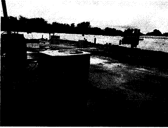
Roof Mounted Condensers | Source: Wynne Real Estate Services (2014)
