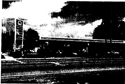
3106 Oxford Street – Marathon gas station
